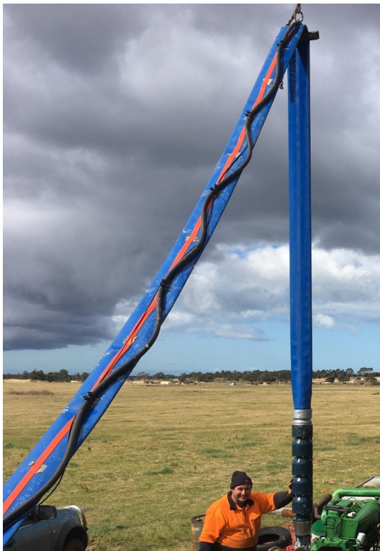
Well-snaked power cable secured with heavy-duty Cable Ties
